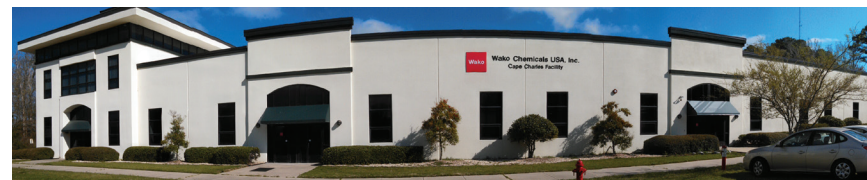
Wako Chemicals USA, Inc. - Cape Charles Bleeding Facility: Cape Charles, Virginia 23310
